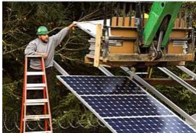
Figure 1: Installing solar panels
